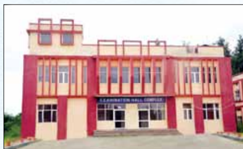
Examination Hall Complex
